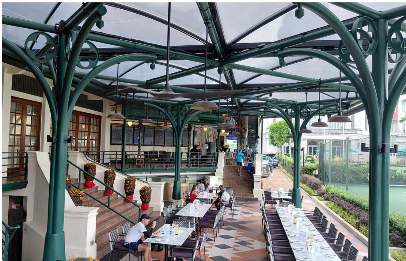
Courtyard Permanent Roofing.
