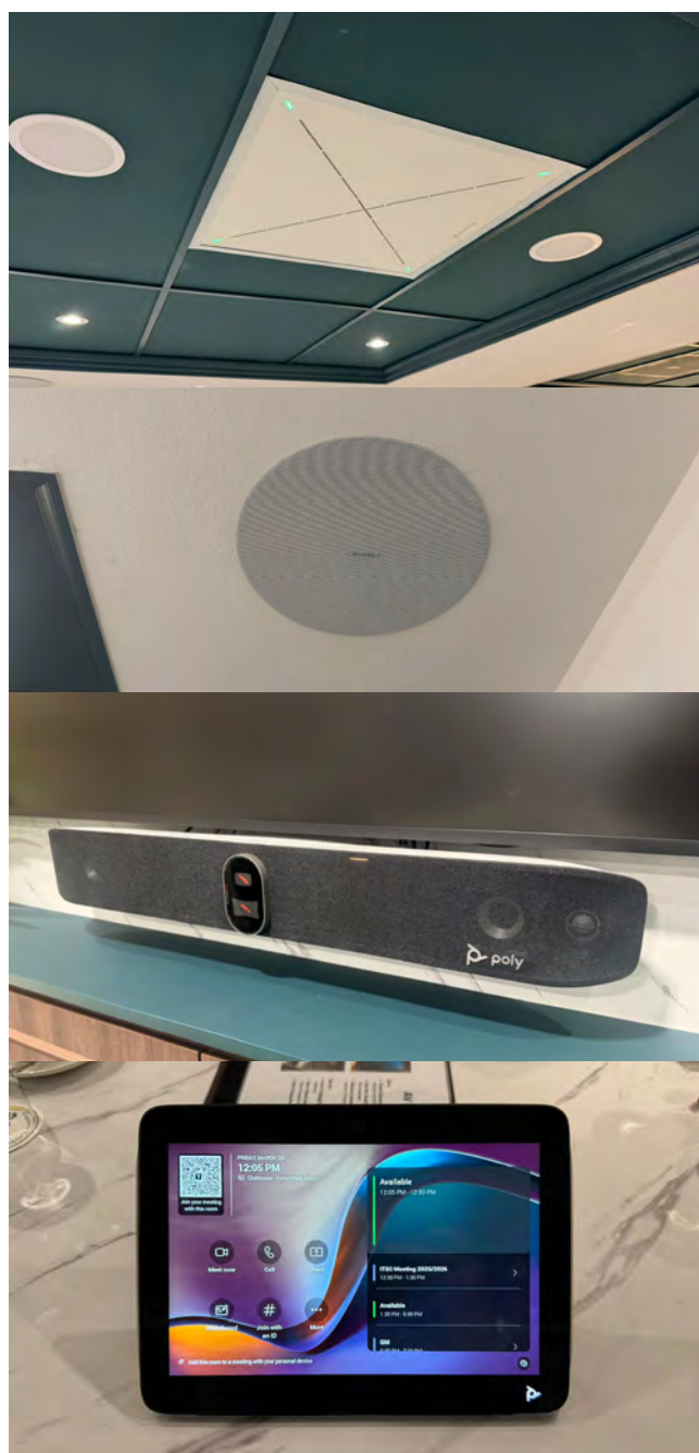
Upgrading the Club Committee Room with modern conferencing systems.
